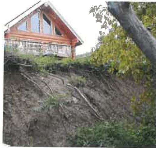
This is an example of eroded bluff in Meeker County.
